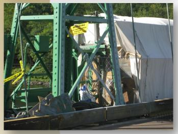
Naik Consulting Group, P.C. (NAIK) performed inspection for structural and bridge deck repairs, abrasive blasting, lead abatement, caulking, and repainting of this structural steel, 585-foot suspension bridge crossing the Delaware River.
